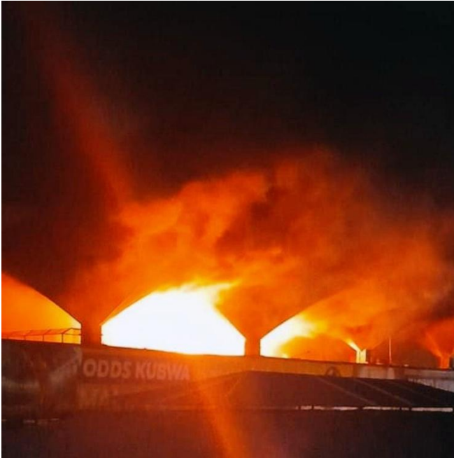
Fig. 4. Kariakoo market in Dar es Salaam – fire outbreak impacts. (Source: Kolumbia, 2021 )
