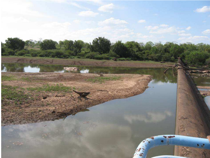
Figure 4.13: A silted weir located at the Prieska
