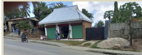
Figure 4:59. Shops along Kilungule road Source: Field survey, 2021
