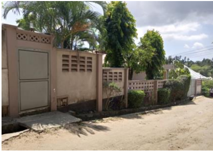
Figure 4:85. Fencing wall with vents in the ‘foreigners’ zone
