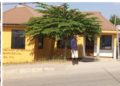
Figure 4:6. Kilungule "A" dispensary. Source: Author field observations, 2021
