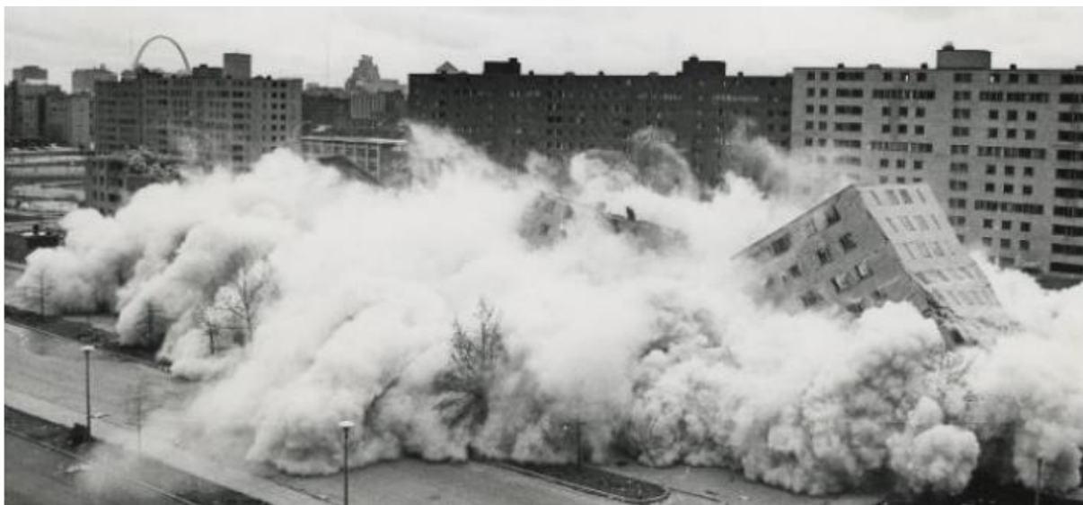
Figure 2:10. Dynamite of Pruitt Igoe in 1971 – 1974
