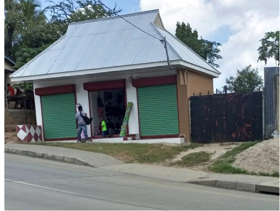
Figure 5:17. New business investments along Kilungule road.
