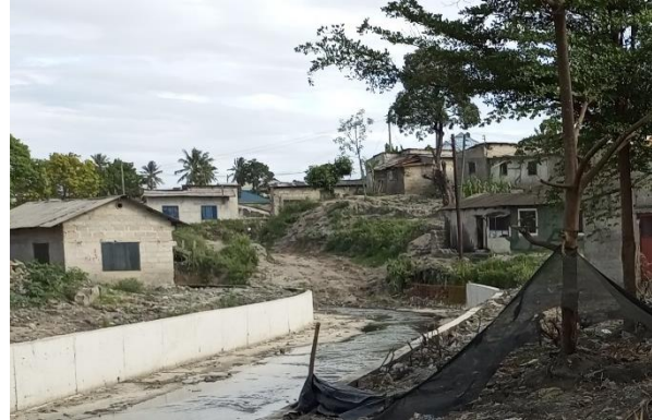
Figure 5:30. New house improvements along the Mpogo River.
