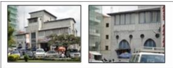
Figure 4 Left Shows the Post Office Building in Totality, Roof Style and Opening Compositions. Right Shows Details Like Pointed Arched Windows with Louvred Shutters, Small Circular Windows, Vertical Elements or Decorations Below Upper Windows, etc.
