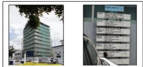
Figure 6 Left is the Building of the Ministry of Constitutional Affairs and Justices, while Right Picture Shows the Building Undergoing Maintenance
