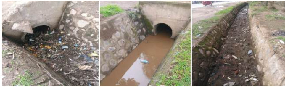
Figure 3. Photographs of the trapezoidal side drain showing (from left to right) the upstream inlet, downstream outlet, and channel approach section
